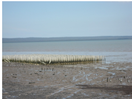
Figure 5. One of three plots at Lang Lang North protected from waves by a “pipe pile field” of ~2 m PVC pipes, established by Hurst (2014).
